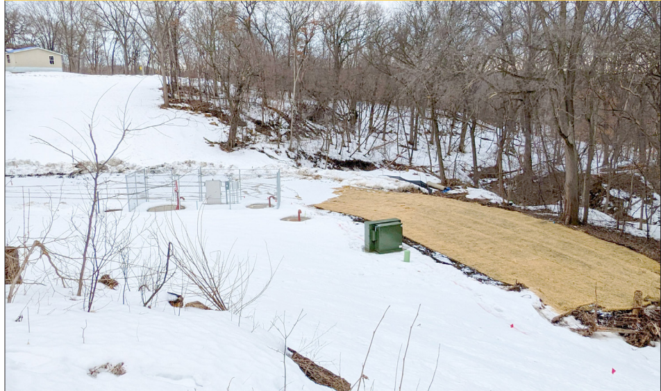
Zumbro Ridge officially connected to municipal sewer service in November 2022. Demolition of the treatment building was completed in January 2023. The yellow erosion control blanket shown in the photo above shows where the old treatment building was. The fences and green service box are part of the new municipal service connection.
